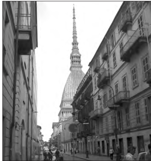
Mole Antonelliana, the Great Synagogue in Torino (Italy), dating from the late 19th century. An imposing public building in the eclectic style. A typical post-emancipation example of a grand and monumental synagogue in the heart of Torino. (Elias V. Messinas Archive)
